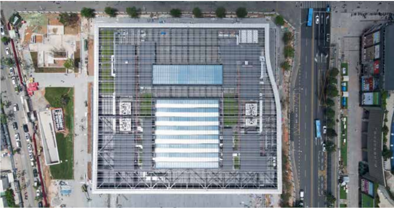
图书馆屋顶景观 View of the library roof
