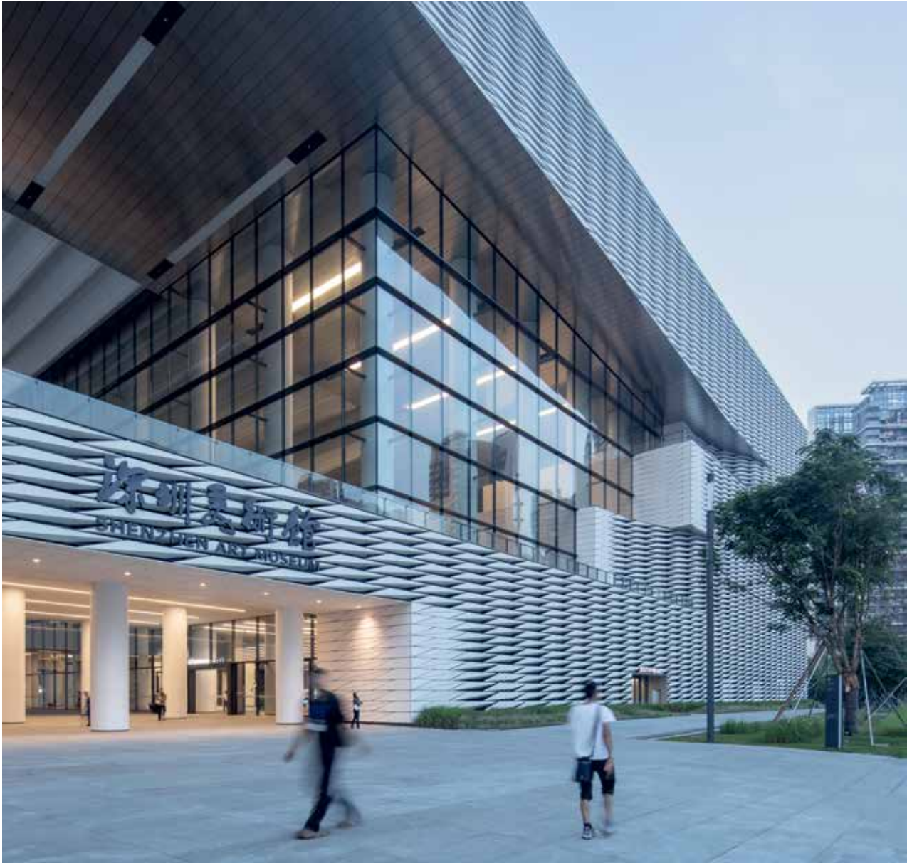
艺术博物馆的入口区域,设有玻璃门厅和雕塑园 Entrance area to the art museum, with the glass-clad foyer and the sculpture garden
