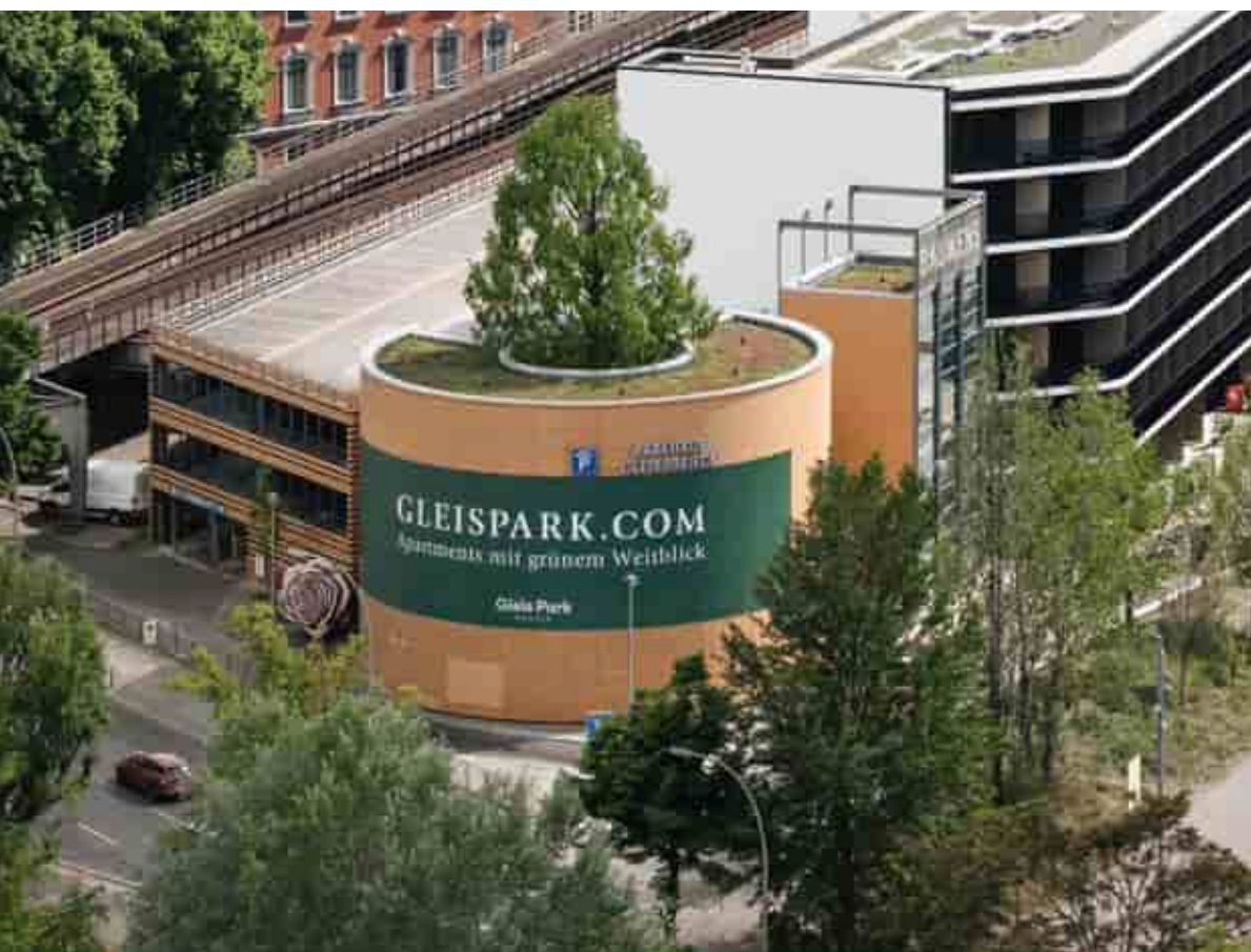
Neubau New Building
