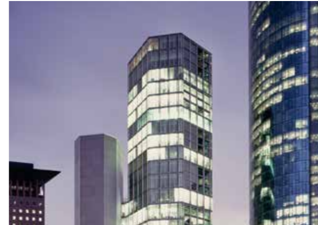
Garden Tower Frankfurt/Main
