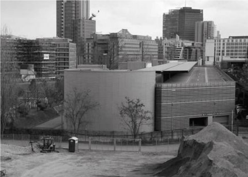
Bestand Parkhaus Building stock car park
