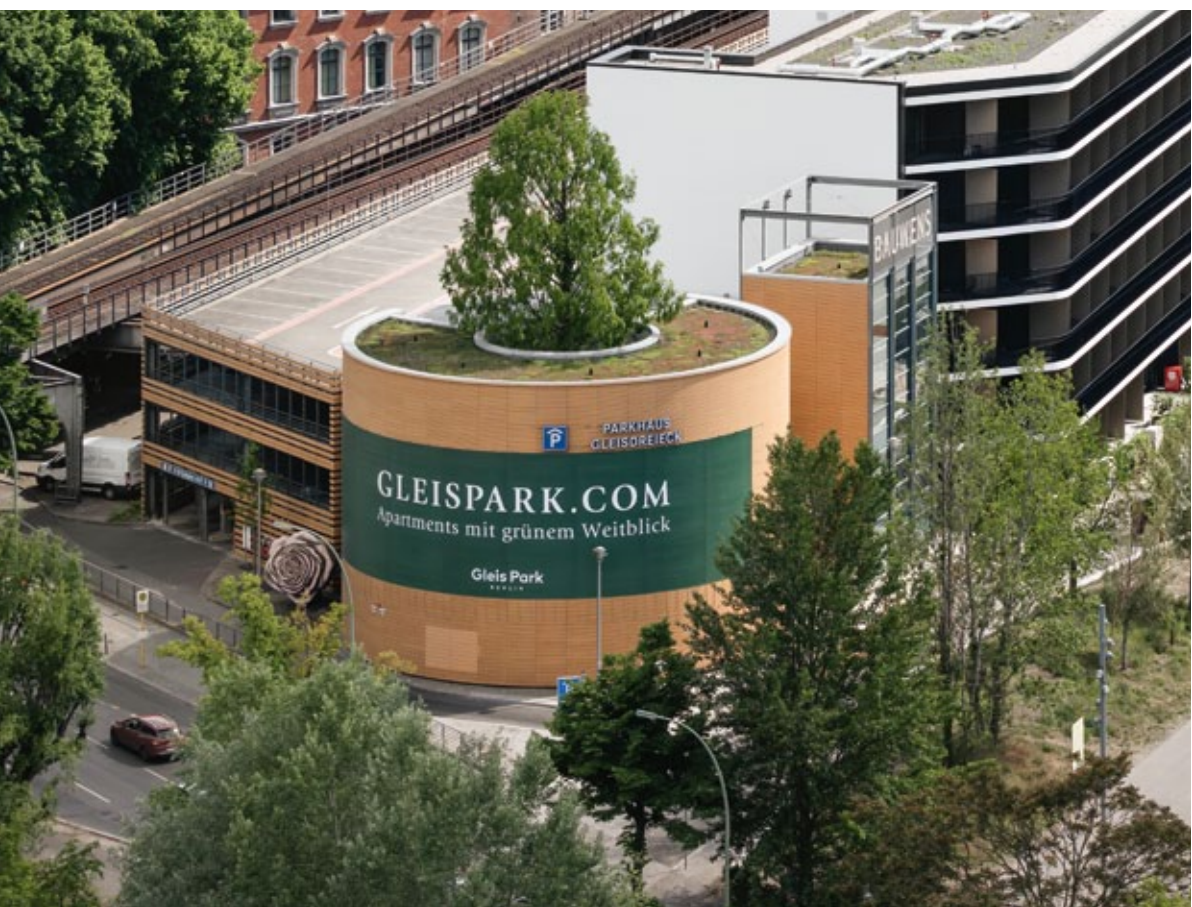
Neubau New Building
