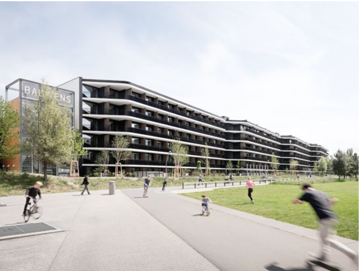
Neubau New Building
