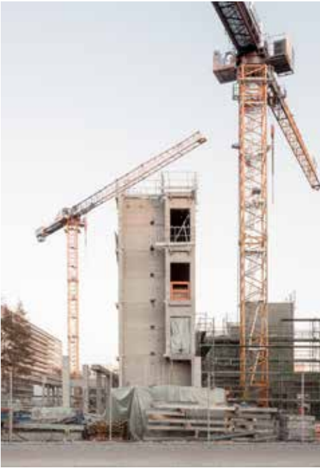
采用预制混凝土构件的系统施工 Modular construction using prefabricated concrete units
