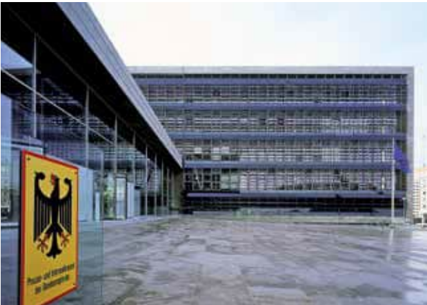
Nordwestansicht Northwest view
