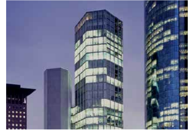
Garden Tower Frankfurt/Main
