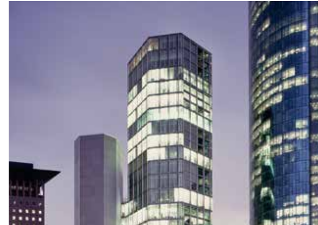
Garden Tower Frankfurt/Main
