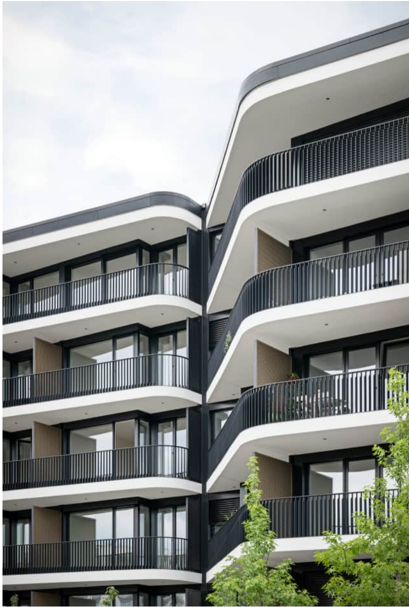
详细视图: 明暗对比构成了立面的结构 Detailed view: Light and dark contrasts structure the façade
