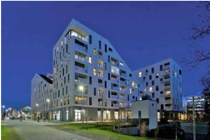
Nordwestansicht Northwest view
