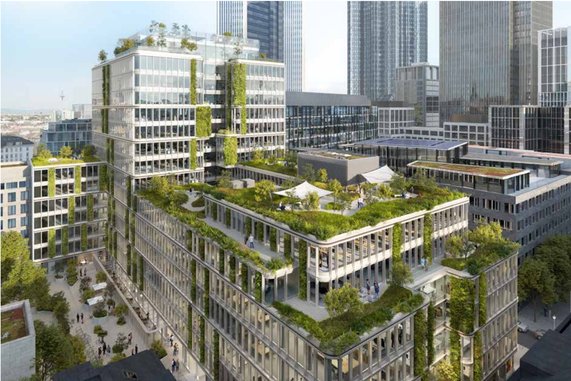
郁郁葱葱的立面绿化、错落有致的屋顶露台以及种植了绿植的内墙，共同营造一个宜居性极高的城市空间。 Lush greenery on the façade, staggered roof terraces, and internal walls covered in plants create an urban space that is a delight to use.
