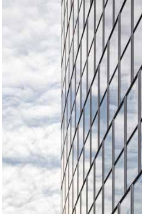
Fassadendetail Façade detail
