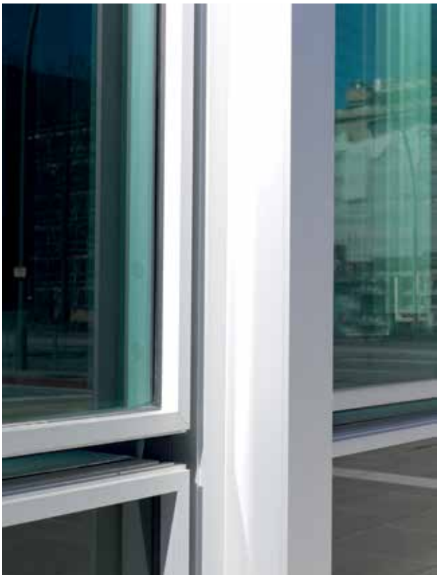
带防撞玻璃和轻金属窗框的箱式窗外观 View of the coffer windows complete with impact pane and light metal frame
