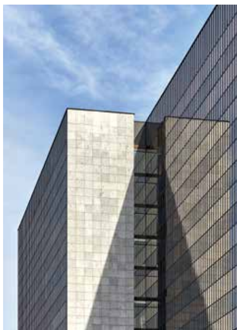
翻新前的阿恩·雅各布森大楼 Arne Jacobsen Building prior to modernization
